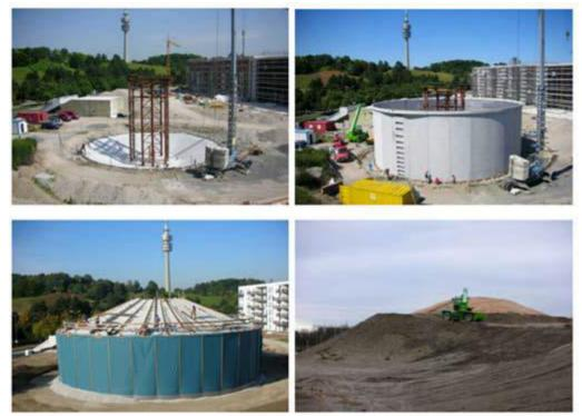
Figure 2 Construction of a tank thermal energy storage system [17]
